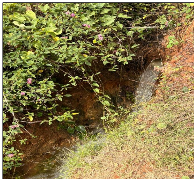
Outlet channel dug at Yaldabhag lake
